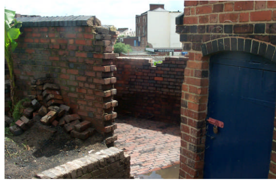
Clean up finished
