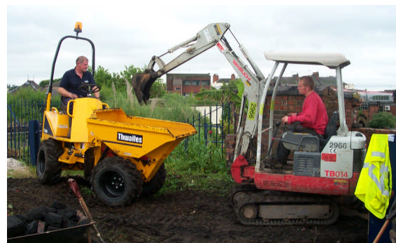
Clean up in progress
